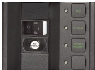
Residual Current Circuit Breaker
